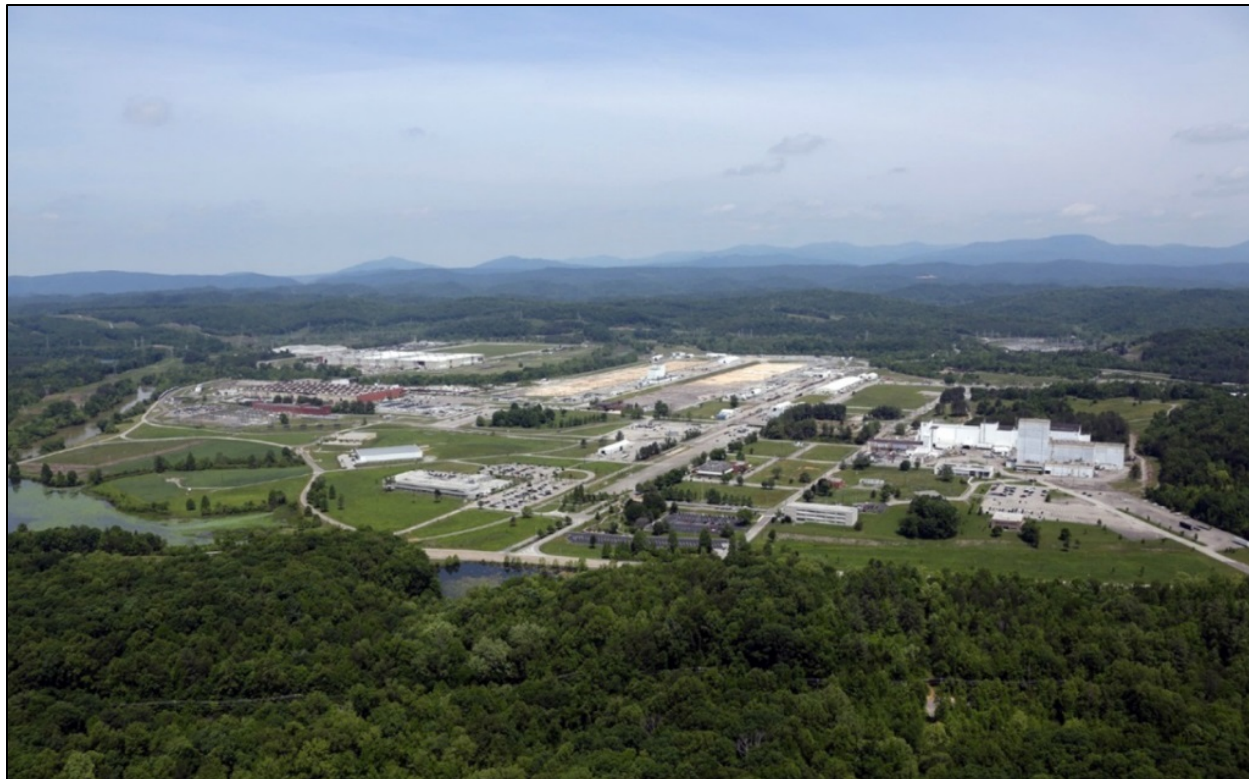
Figure 1.8. Aerial view of East Tennessee Technology Park
